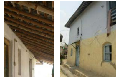
Figure 2 Roof with slates and adobe walls
